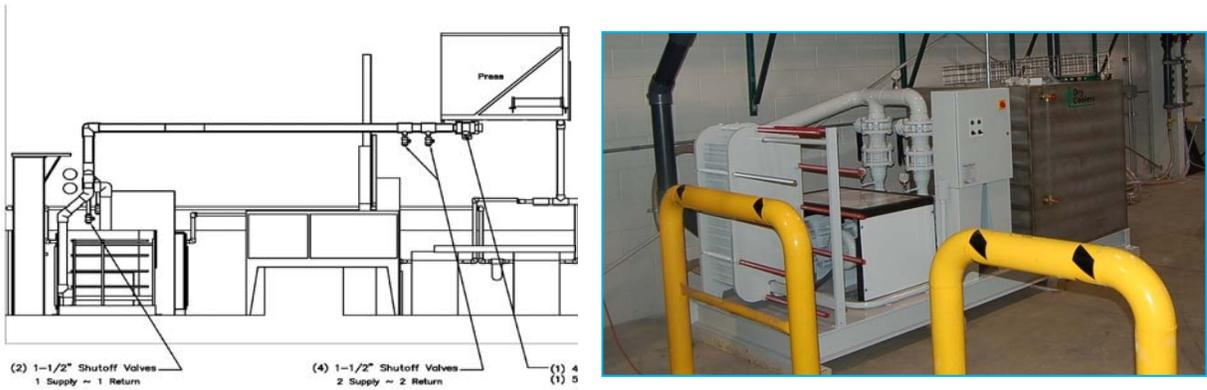
Figure 43. Schematic and picture of the coolant system for delivering coolant to the coil and the power supply
